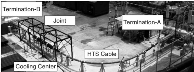
**Photo 5.** Completed 30-meter HTS cable system
